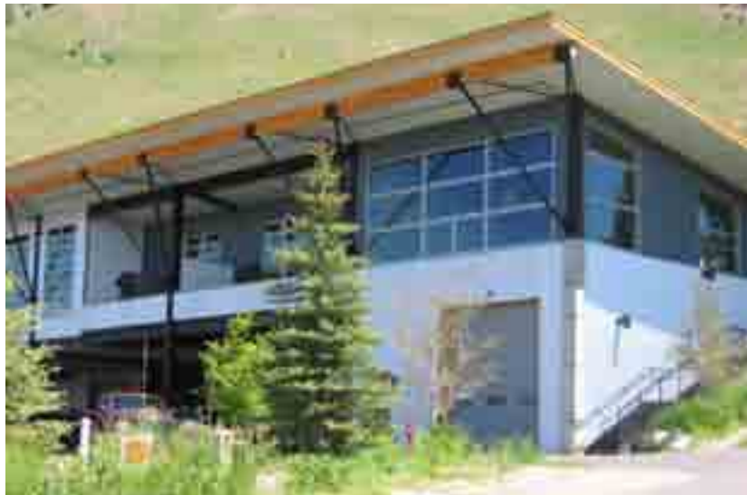
The Elk Avenue Condos, located in the South Park Business Park, include six accessory residential units on the second floor of the building.
