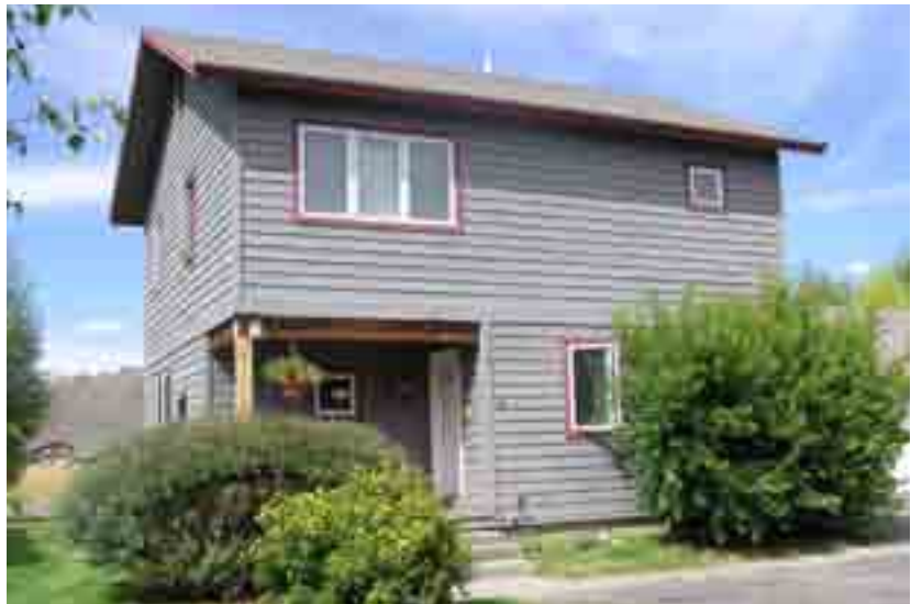
Mountain View Meadows home. First deed restricted affordable housing neighborhood. Photo courtesy of Jackson Hole Community Housing Trust.
